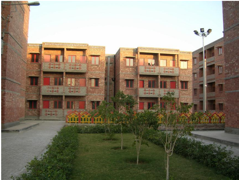
Figure 1: Example of a residential complex at Bawana Estate, illustrating the use of pre-cast columns, filled with conventional bricks, used in a mass housing development for industrial workers. It is possible to complete a complex in a very short time using the pre-cast and monolithic systems (as little as 4 months for one block within a multi-complex development). Sale prices vary depending on the size of the unit, e.g. single unit : 16\text{m}^2 = \text{US } \$ 2200 (approx.); double unit : 31.93 \text{ m}^2 = \text{US } \$ 4500 (approx.); 3 roomed unit : 40\text{m}^2 = \text{US } \$ 6300 (approx.) Materials are available at low cost and greening is used extensively.
