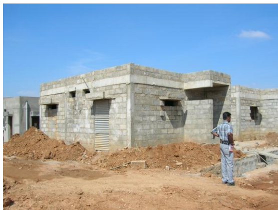
Figure 6 : Low income housing under construction
