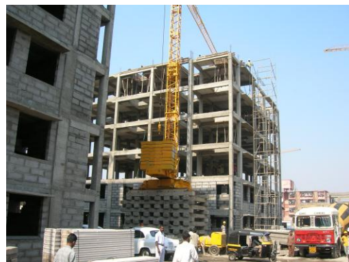
Figure 10 : Transit area under construction Mumbai
